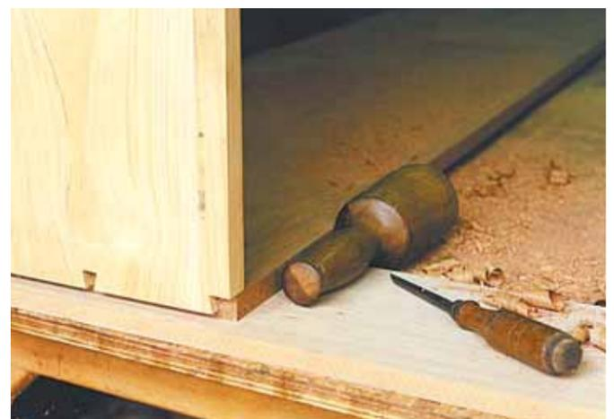
Dovetailing with mallet and chisel
