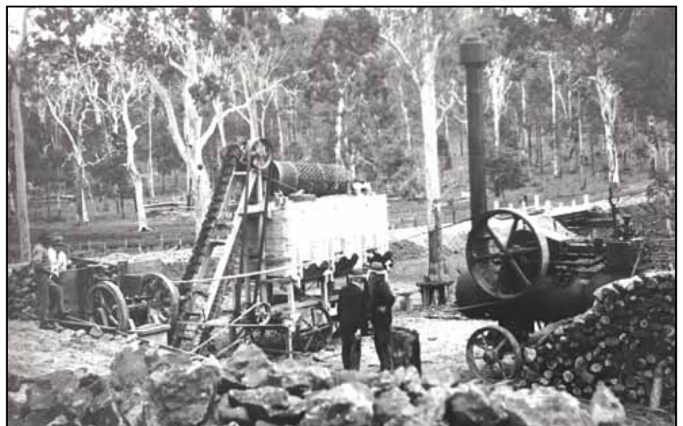
Road construction, stone grader, c1925.
